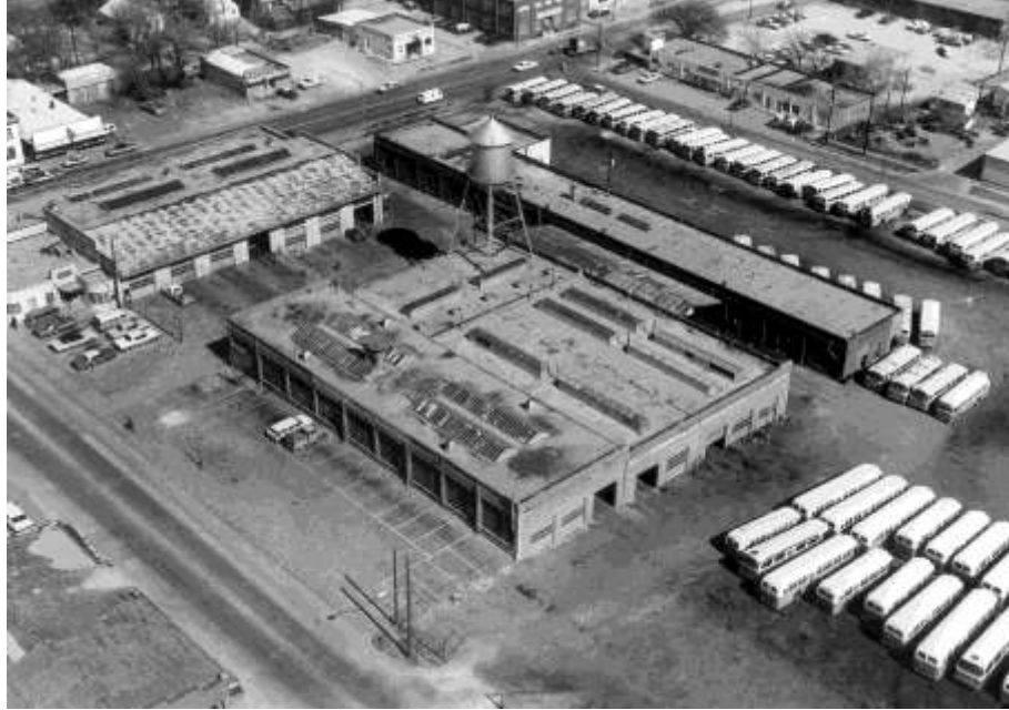
Original T facility at 1600 E. Lancaster
