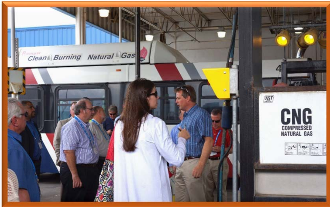
The T provided technical tours for the guests at APTA. This is the CNG fueling center at The T.
